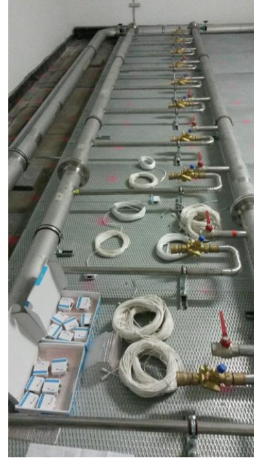
Waterleak Detectors HWg-WLD at Biozentrum University of Basel
